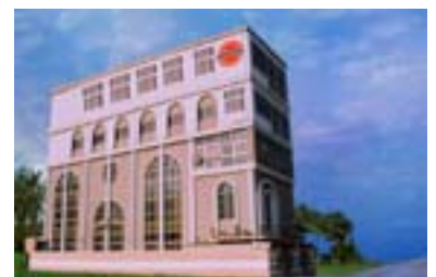
Production - Inductive Components
