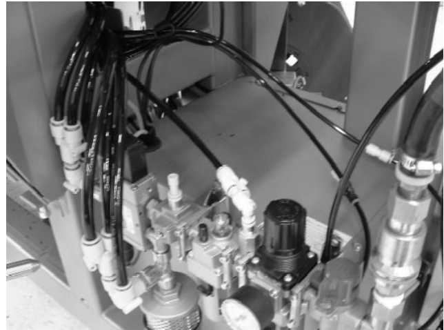
Plumbing Prior to Installation Figure 6
